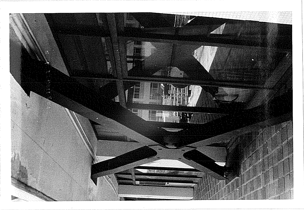
Fig. 1.3.1 Sendai School, Japan; steel bracing retrofitting
